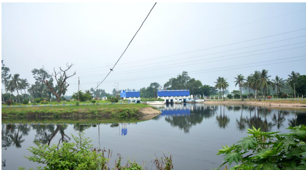
A sewage inflow barrage gate at Bantala, EKW
